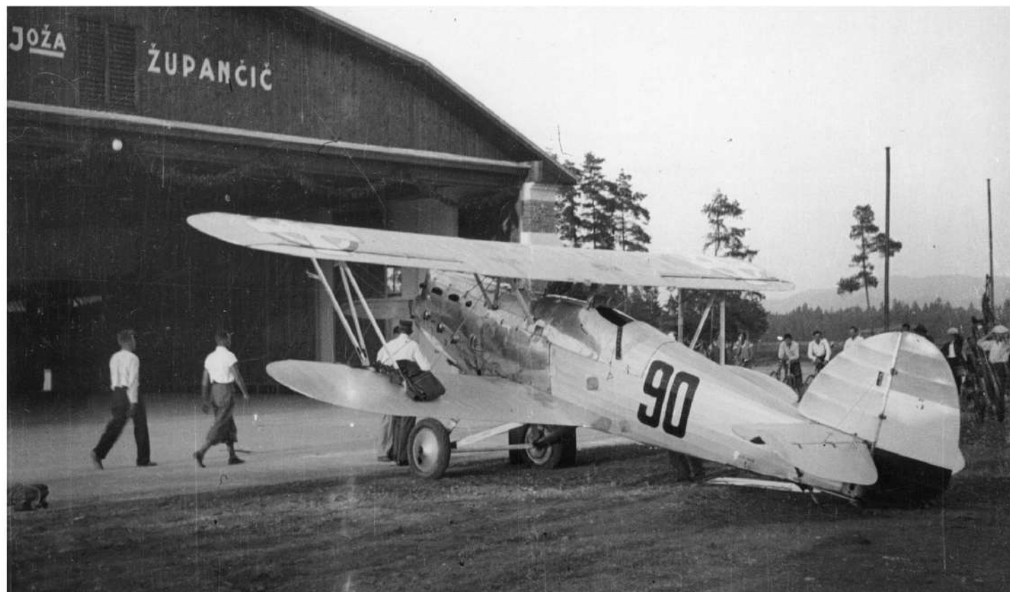
Hispano - Suiza (HS 12Nb) powered Hawker Fury Mk.I, now officially as the VVKJ №3, photographed in Slovenia at the Ljubljana airport and in front of the "Major Joža Župančič" hangar. The reason for installing the Hispano engine was the great pressure by the French on the Yugoslav Government to buy at least their engines for the new fighter planes. Later this aircraft was sent back to Hawker for a reinstallation of its original Rolls-Royce engine. (Marko Malec)
